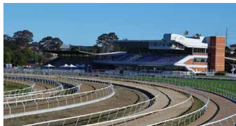
Upgraded Fast Sand and new PVC rails Fast Sand and Trotting Tracks
